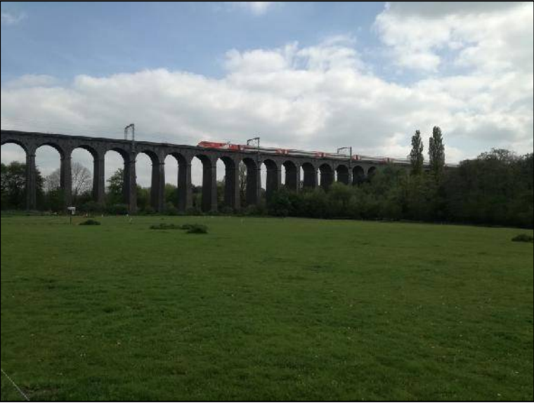
View of Welwyn / Digswell Railway Viaduct
