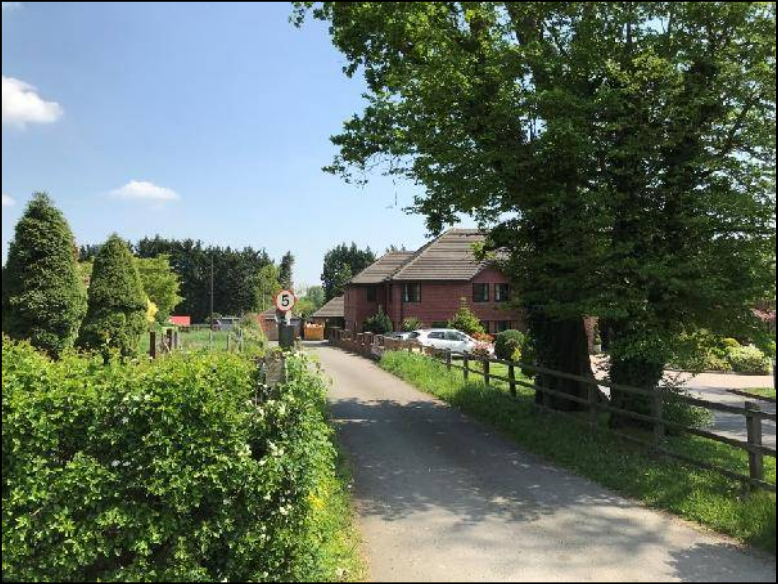
Care home alongside the B197 Great North Road.
